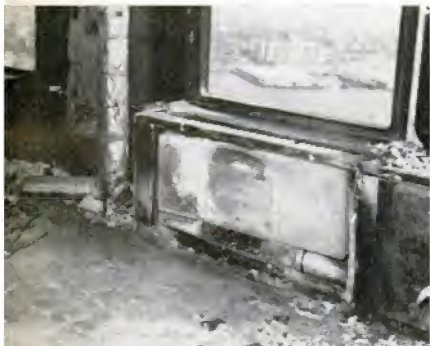
BURNED-OUT FLOOR of Plaza building reveals that "fireproof" materials do burn. Fire was traced to ceiling area.
